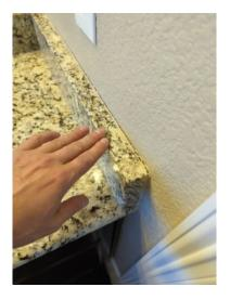
The countertop was missing sufficient caulk/sealant at the wall or sink. This can lead to water damage. I recommend adding sealant at sides and corners where counters touch walls and sinks. Here is a helpful DIY video on caulking gaps.
