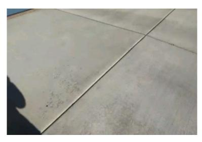
Concrete surfaces are weathered and deteriorated. I recommend repair or replacement by concrete professional when the driveway or walkway looses its functionality.
