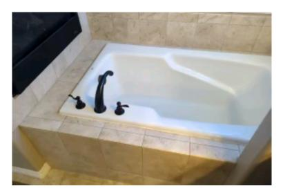
At the time of inspection I observed a soft whistling noise coming from one of the fixtures in the home. This is typically the result of some air in the supply line. Sometimes it will work its way out on its own, but if the problem persists, I recommend evaluation by a licensed plumber in any repairs to be made.
