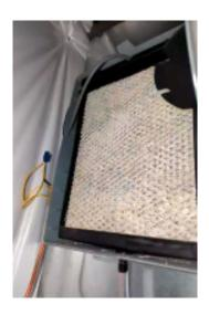
The humidifier had excessive mineral deposits at the time of the inspection. Recommend replacing the pad.
