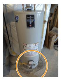
Water stains were observed beneath water heater, indicating a past or present leak. Recommend further evaluation and repair by a qualified plumber if necessary.
