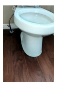
The toilet was loose at the base. This may be from a damaged flange or a failed wax seal. In any case, this should be remedied before a leak occurs.
