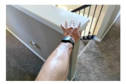
I recommend securing the handrail.
