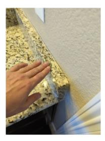
The countertop was missing sufficient caulk/sealant at the wall or sink. This can lead to water damage. I recommend adding sealant at sides and corners where counters touch walls and sinks. Here is a helpful DIY video on caulking gaps.
