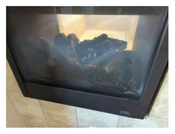
The glass on the gas fireplace was foggy at the time of the inspection. Recommend cleaning of glass.
