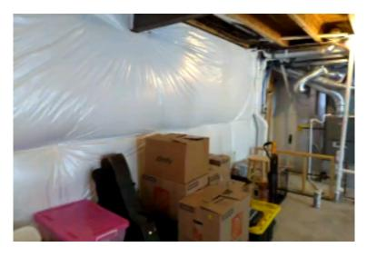
Foundation basement or crawlspace walls were finished and/or insulated at the time of inspection. Only walls which were fully exposed could be thoroughly inspected for structural deficiencies.
