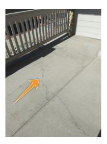
I observed some minor cracks in the cement. This is very typical due to soil movement. I would consider these cracks cosmetic, but I do recommend using a sealant to prevent water intrusion. Monitor and maintain as necessary.
