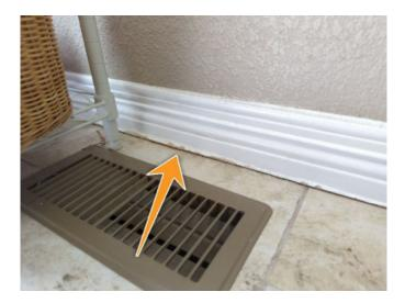
There was minor damage to one or more pieces of trim at the time of the inspection. Recommend repair or replacement.
