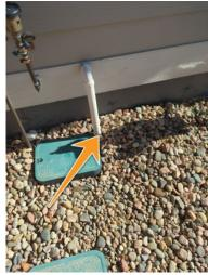
I was unable to view where the sump pump discharge terminated. It is buried beneath the front porch and I was unable to find where it ends. Recommend asking seller pertainant information regarding sump pump discharge.
