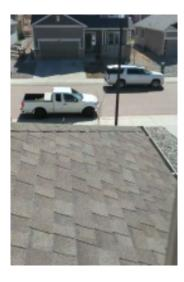
At the time of inspection there was some mechanical damage present on the roof covering. This is damage that's not attributed to a storm or hail. It is often the result of a contractor walking on the roof and scuffing the shingles. Mechanical damage typically does not affect the roof's ability to shed water. If there are further concerns I recommend having a licensed roofer evaluate.
