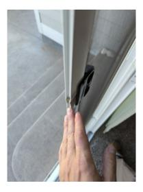
The sliding glass door screen appears to be damaged. Recommend repair or replacement.
