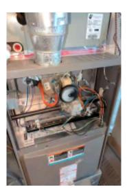
The furnace is dirty. I recommend servicing by a qualified HVAC technician.
