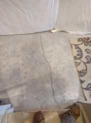
There is evidence of typical cracking in the basement concrete slab. Recommend sealing the cracks and monitoring for further movement.
